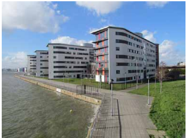
University of East London dockside buildings © Rory Walsh
