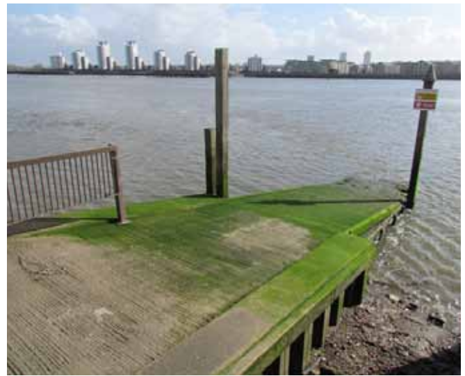
Bargehouse Road slipway © Rory Walsh
