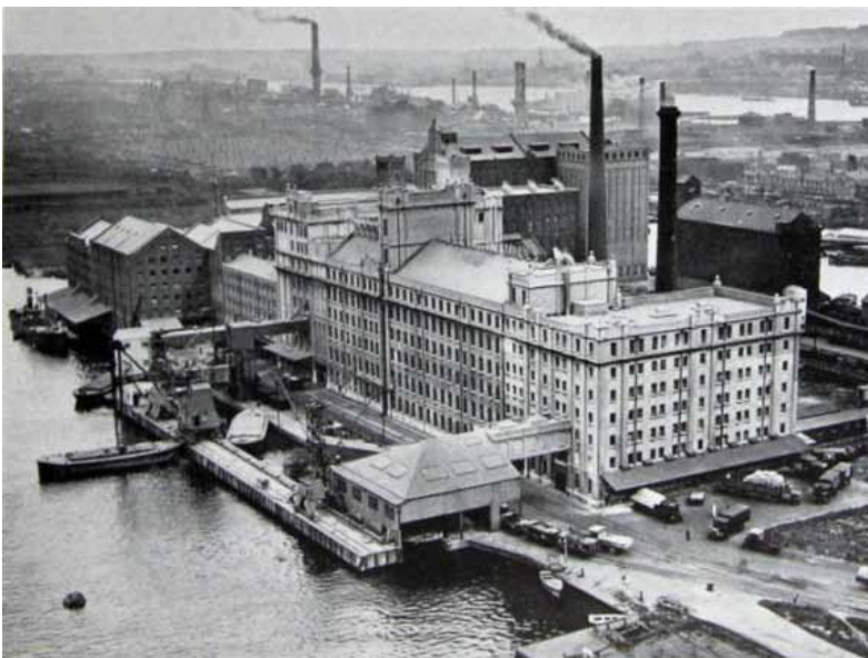
Spillers Millennium Mills beside Royal Victoria Dock (1934) Wikimedia Commons (CCL)
